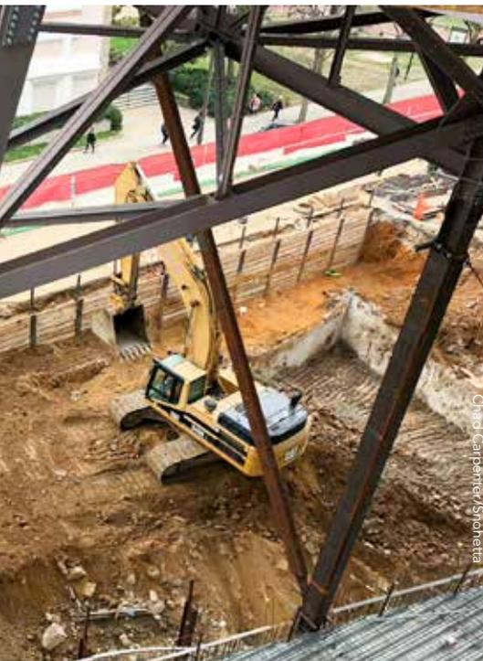
below: Truss erection at the southwest entrance. The corner column at the far right is a temporary support.
